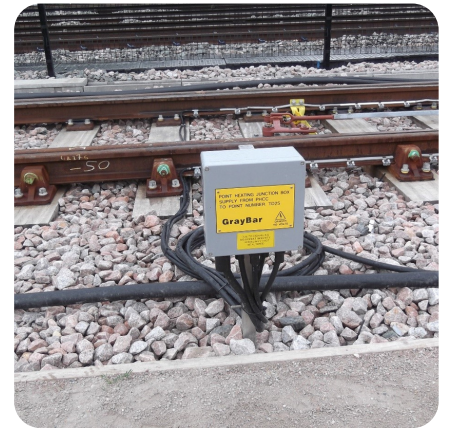
Trackside Junction Box
