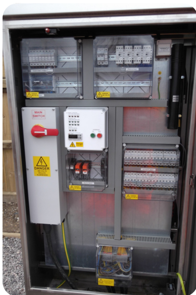
GrayBar Cubicle - interior
