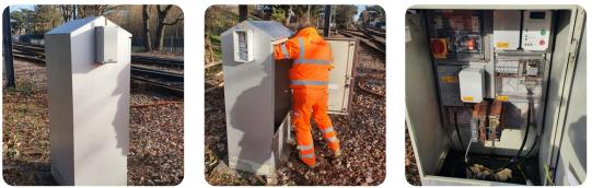
Using IP66 GRP Weatherproof Enclosures, these have been fitted to a number of cubicles on the Network, to allow them to continue to function and extend the working life of the Cubicles.
