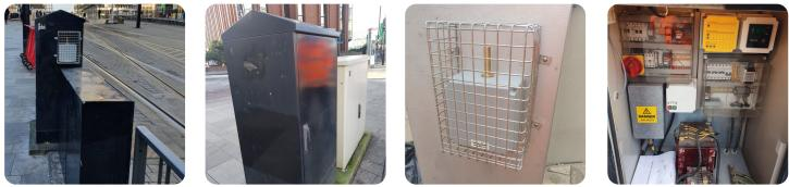
These Temperature Probe housings are aluminium and are also further protected by a Hot Dipped Galvanised Cage, giving added protection and security for cubicles situated in the busy urban centre of Croydon.
