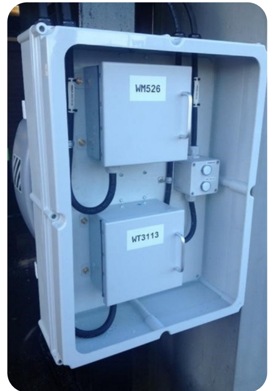
Watford Junction - GBK4013 - RA Indicator Station, Twin
