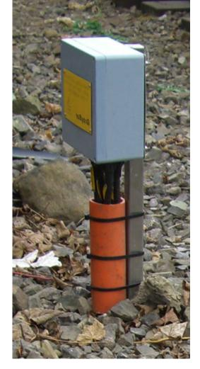
Mounted onto a 3mm Thick, Grade 316 Mechanically Abraded Stainless Steel, Plate and 40mm square section post.
